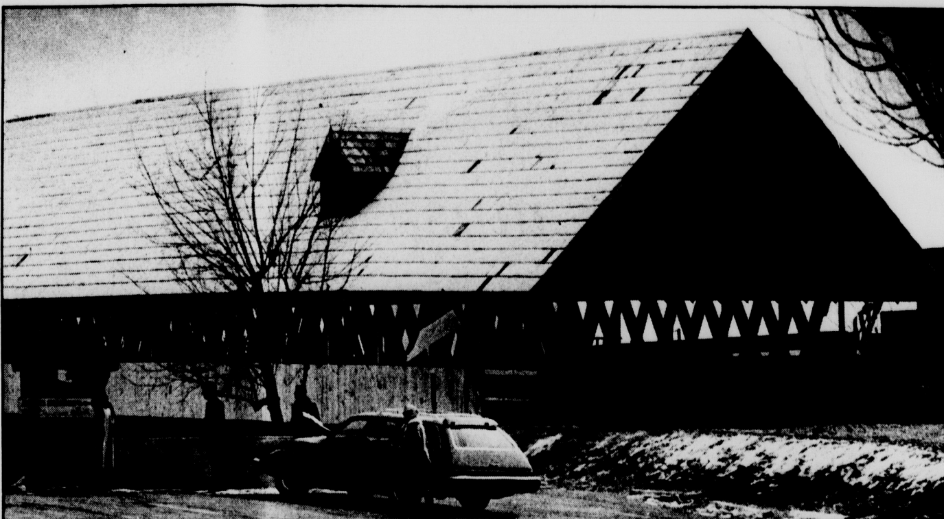
It took a team of oxen to do it, but Frankenmuth, Mich. finally has its famed wooden covered bridge in place on the west bank of Cass river there. The 230-ton, 239-foot structure was built on dry land and pulled by the oxen four hours a day for 12 days. The bridge is expected to be open to traffic this summer and dedicated in the fall.
