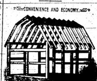
FIALLS SELF-SUPPORTING RAFTER Gambrel and Mansard Roofs. PATENTED, APRIL St. 1975-4
