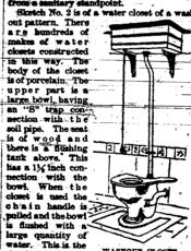
It is carried on bracke bowl of porcelain ware. It has a standing over flow at the back and inside of the bowl, this bowl baving a straight back rather the true semi-spherical form, as is common.
