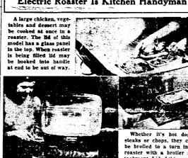
be broiled to a turn in a oaster with a broiler at tachment. Lid of this roast-er has sliding-cover vents to control the air circula-tion for browning fowls,
