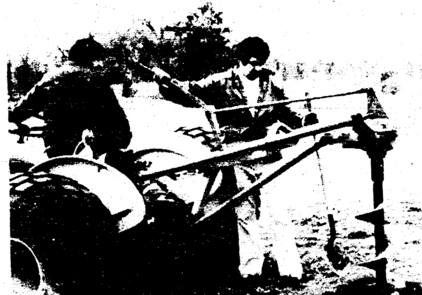
Dave Wilson and Jim Schook used Dave's tractor to dig the holes for the trees.
