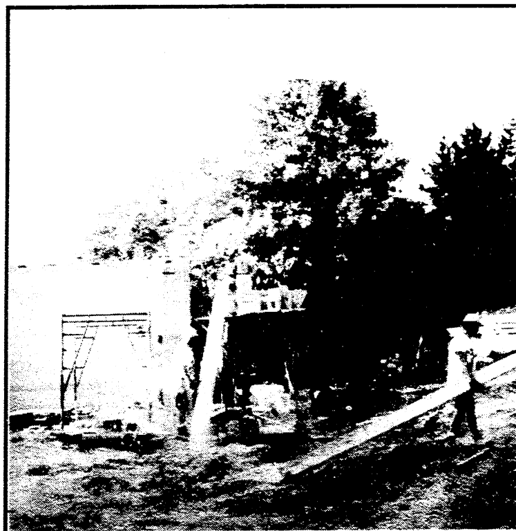
The work on "Phase Two" continues
