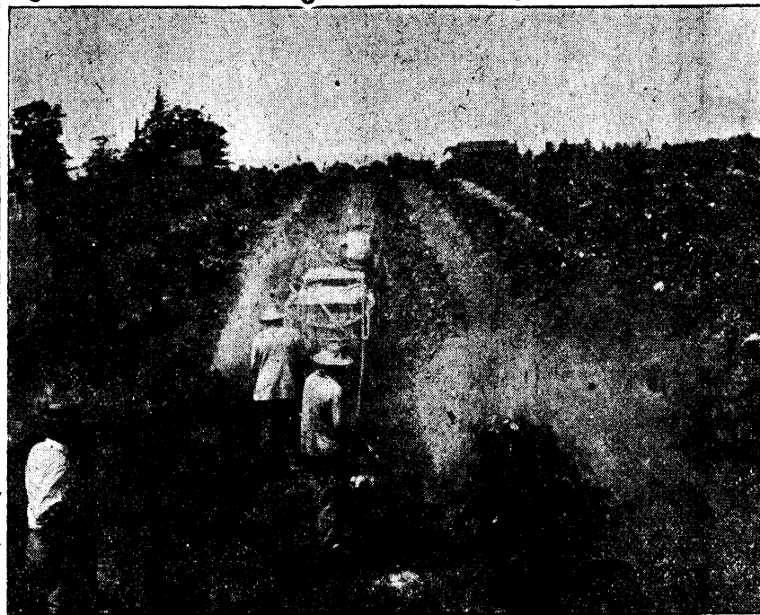
The "trailer" system of vineyard spraying. Two men are required to handle the nozzles, but a more thorough coverage is given.
