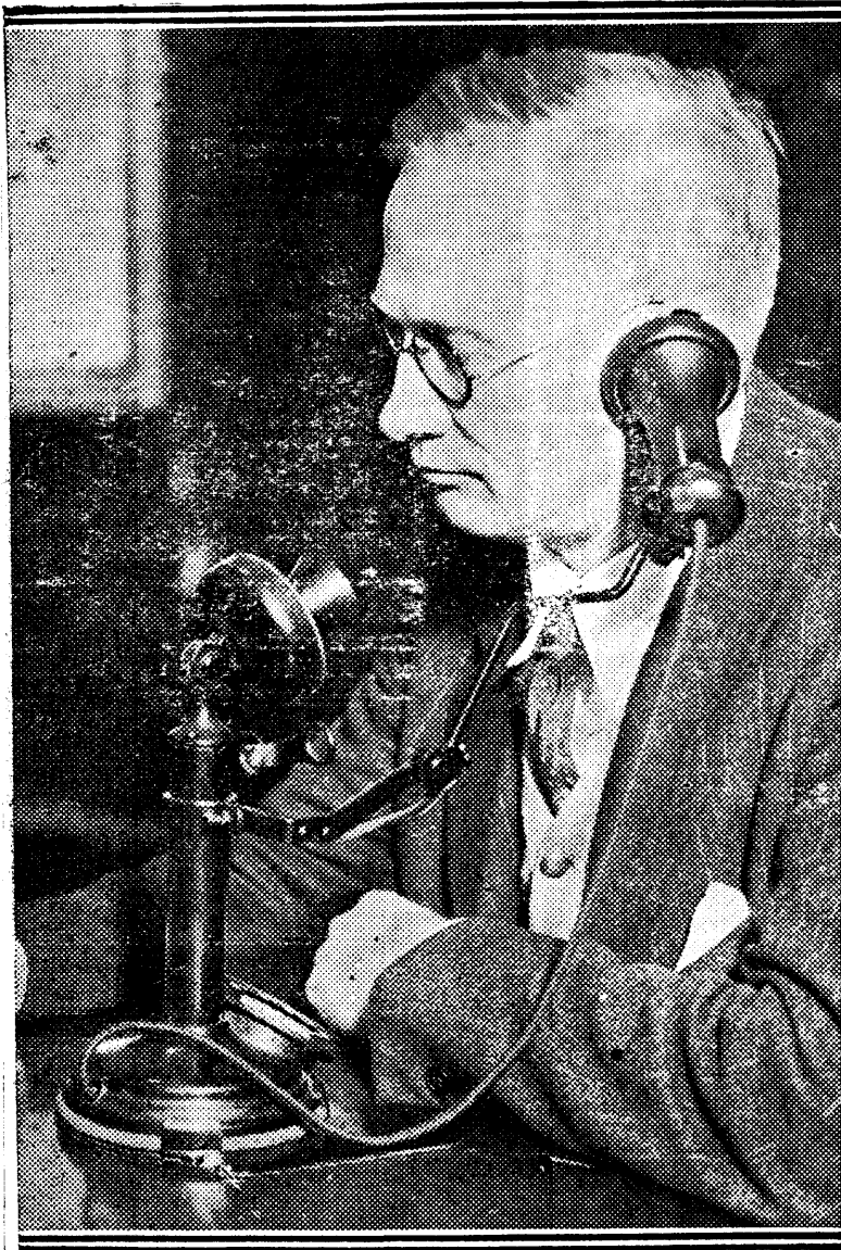
An invention is said to make it possible to have both hands free while telephoning. It automatically holds the receiver to the ear. N. C. Hill is demonstrating it in New York.
