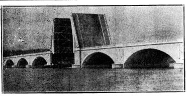
The new Arlington memorial bridge, which spans the Potomac River and connects the beautiful national cemetery with the city of Washington proper, has the largest draw span in the world. Each span weighs 6,000 tons and is raised to a 65 degree angle when opened to allow vessels to pass through. Despite the great weight the spans take but five minutes to open and close.
